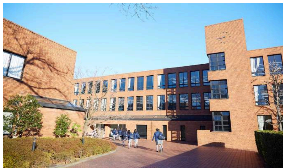
A building of St. Hilda's School
