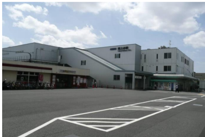
Current Sakurajosui Station / Photo by Ryoma Noguchi
