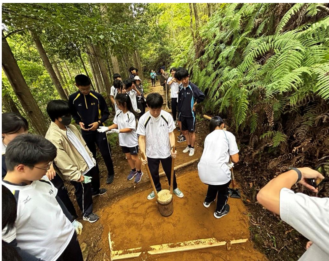
(left) Students used traditional tools called “tako” to harden the ground. (right) Students collect soil to repair the mountain road.
