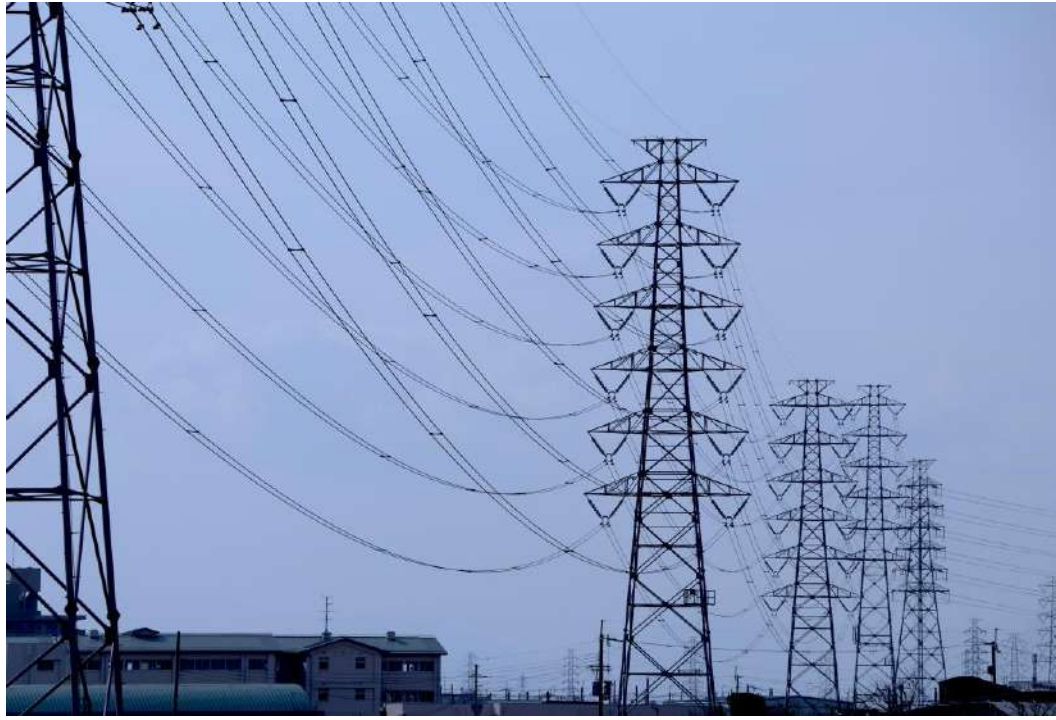
Electricity is transferred through high-voltage transmission line of over 300,000 volts.
